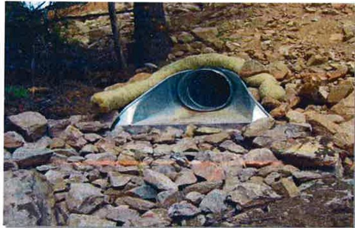
Photograph TOP-1. Riprap outlet protection.
