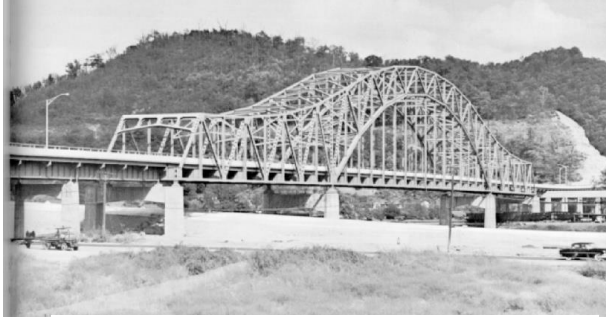
Figure 1: The Charles Yager Bridge located on the West Virginia Turnpike.
