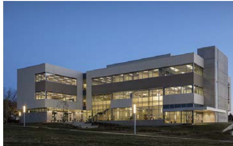
Remediation of the General Classroom Building
